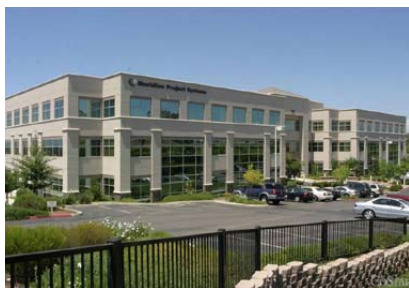
Calpine, a leading geothermal power producer, will occupy 40,000 square feet of space previously occupied by Meridian Project Systems at 1180 Iron Point Road in Folsom.
